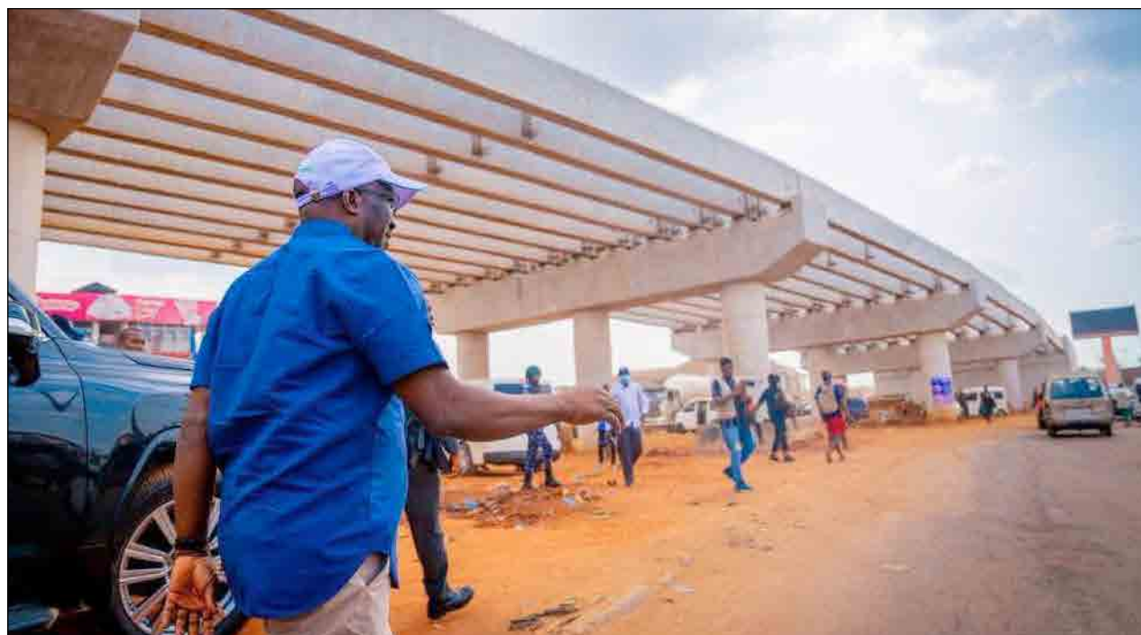
INSPECTING FLYOVER PROJECT:
