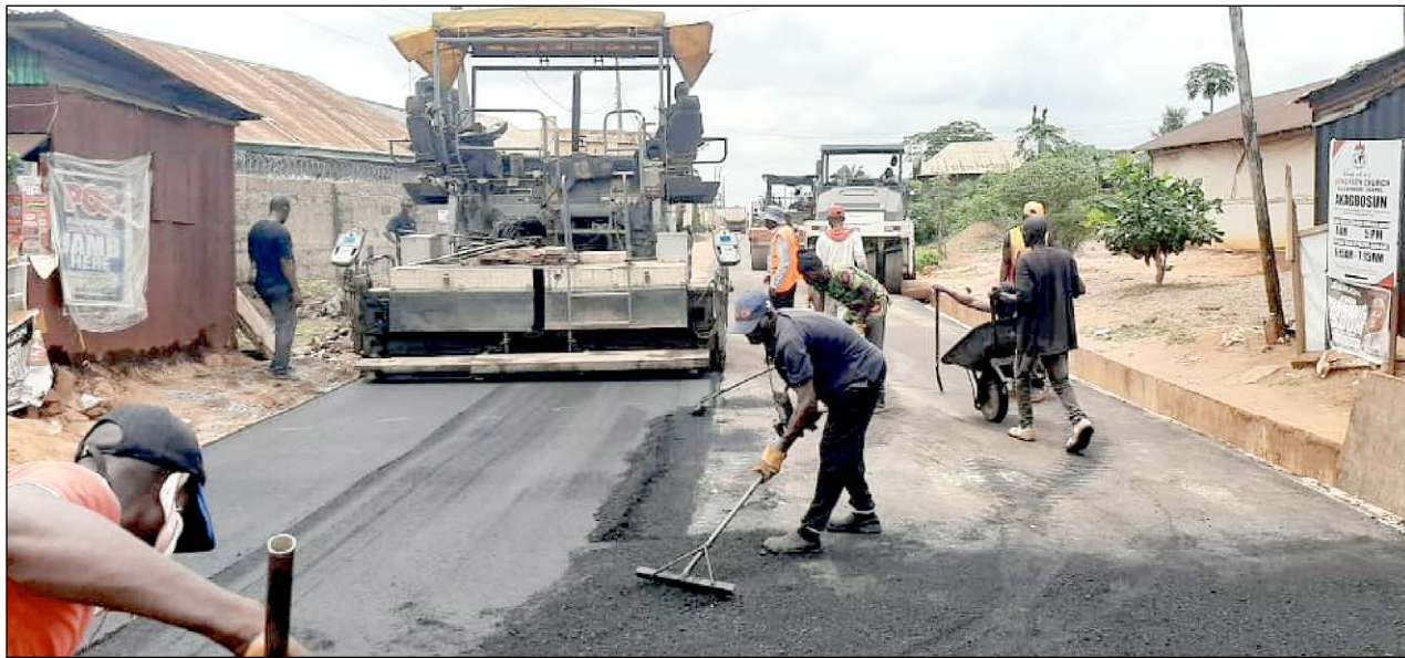
EKEHUAN ROAD: Asphalt Laying on Ekehuan Road, Benin City
