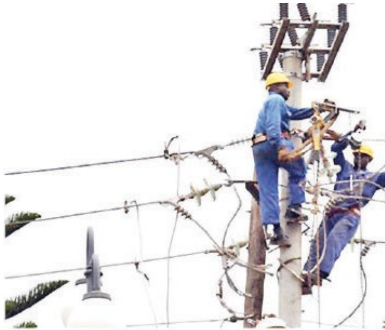
Officials working on electric lines.
