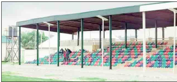
BWARI TOWNSHIP STADIUM
