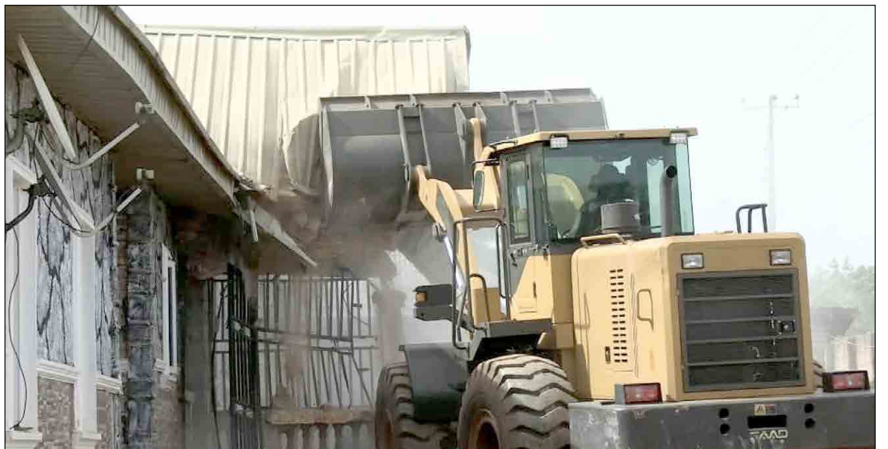
DEMOLITION IN UBIAJA:
