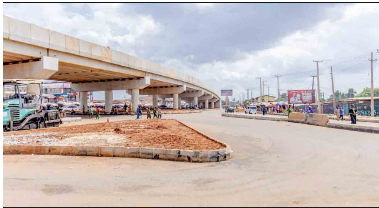
FLYOVER: Ramat Park flyover
