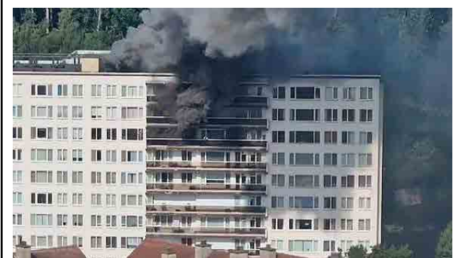
Fire at Antwerp apartment block
