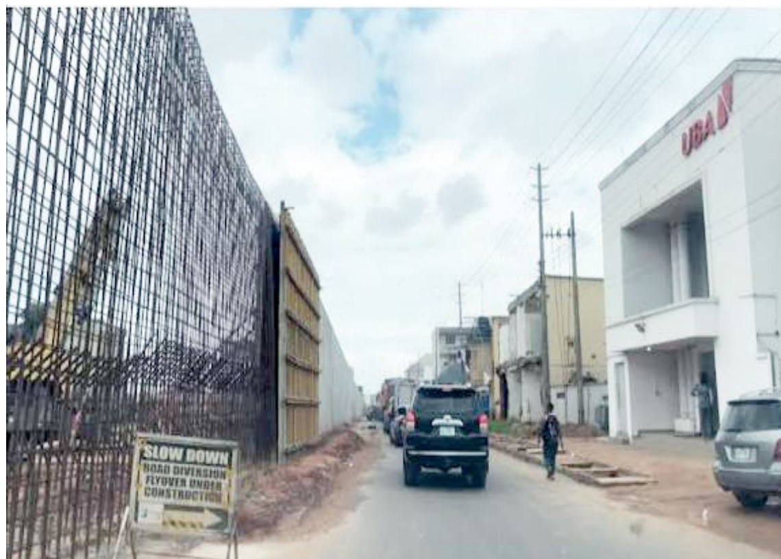
ONGOING CONSTRUCTION OF THE ADESUWA FLYOVER BRIDGE
