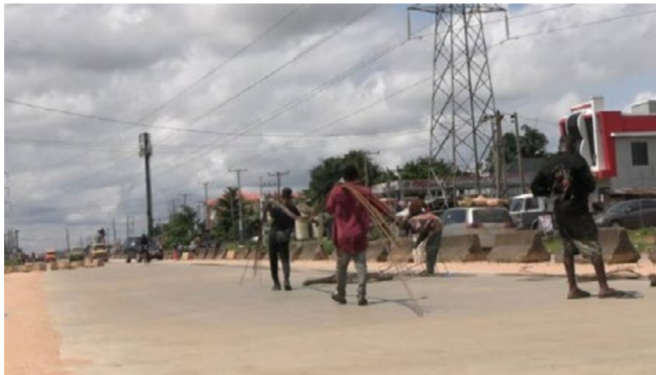
Federal Roads in Edo under construction
