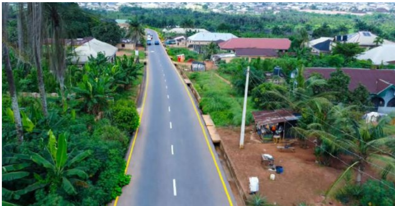
ROAD INFRASTRUCTURE DEVELOPMENT: Iwogban - Ute axis in Benin City.
