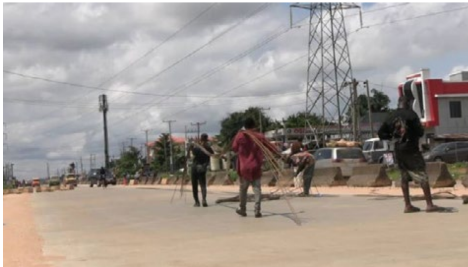
Federal Roads in Edo under construction
