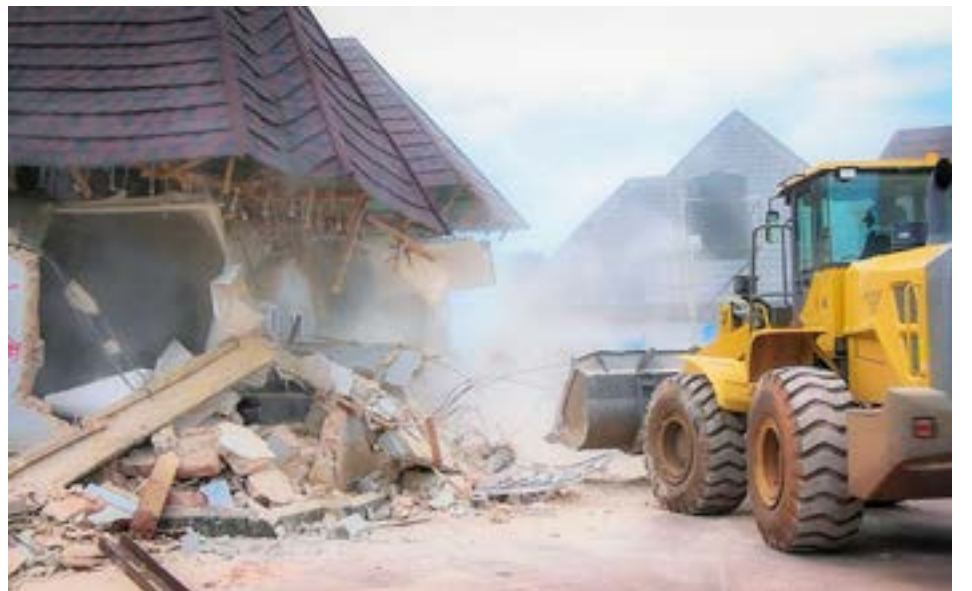
Demolition of the building by the taskforce
